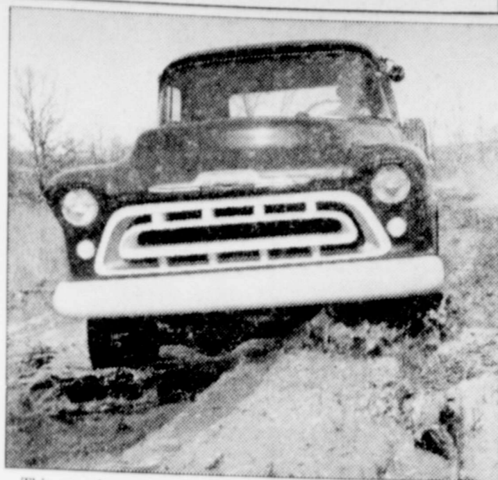
This new four-wheel drive Chevrolet truck plows through hub-deep mud with power and traction to spare. (Note the offset front drive axle under the bumper at the left.) Designed for difficult off-road operations on steep grades, rough terrain, and in deep sand and mud, this all-wheel drive unit now is in production. It is available in 12 models including the suburban carryall; 3/4-ton, 1-ton and 1-ton pickup; 1-ton panel; 3/4-ton and 1-ton stake.
