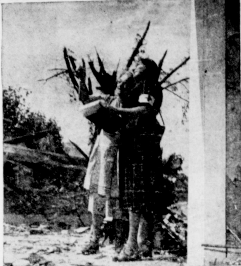
BLACKWELL, OKLAHOMA—Mrs. Bertha E. Kubly, 2 South Street, Worcester, Mass. (right) plans rehabilitation for Mrs. Flora Parr, age 71, whose home was completely demolished in the tornado which struck the community May 25th. Because of her long experience in all phases of disaster work, Mrs. Kubly was flown to Blackwell. She said, after visiting the ruins of the Parr home and Blackwell in general, "We thought the destruction in the Worcester tornado of 1953 was bad but it cannot compare to what I have seen here." (ARC Photo by Palmer)
