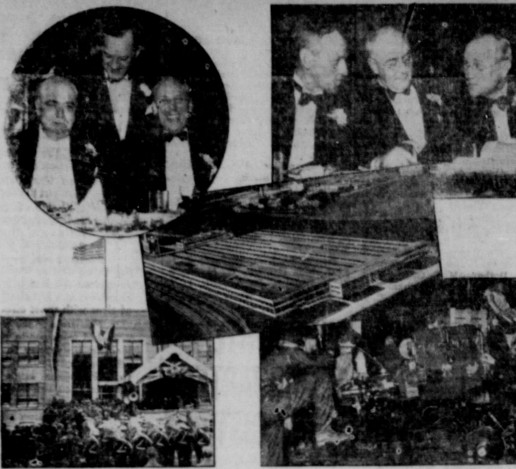
Governmental, state and civic officials joined with the principal executives of General Motors Corporation in the formal opening of the new 80,000-car-a-year Chevrolet assembly plant in Baltimore recently. The new plant (center) was dedicated with impressive ceremonies (lower left), and Chevrolet, Fisher Body and General Motors officials were guests of the Baltimore Association of Commerce at a formal banquet in the evening. W. E. Holler, vice-president and general sales manager of Chevrolet, is shown (at center) with Maryland's Governor, H. W. Nice, and Alfred P. Sloan, Jr., president of General Motors (upper left). M. E. Coyle, president and general manager of Chevrolet, is pictured in the upper right photo with Senator Tryding (left) and Mayor H. W. Jackson, of Baltimore (right). Lower right shows the first motor car built in that city.
