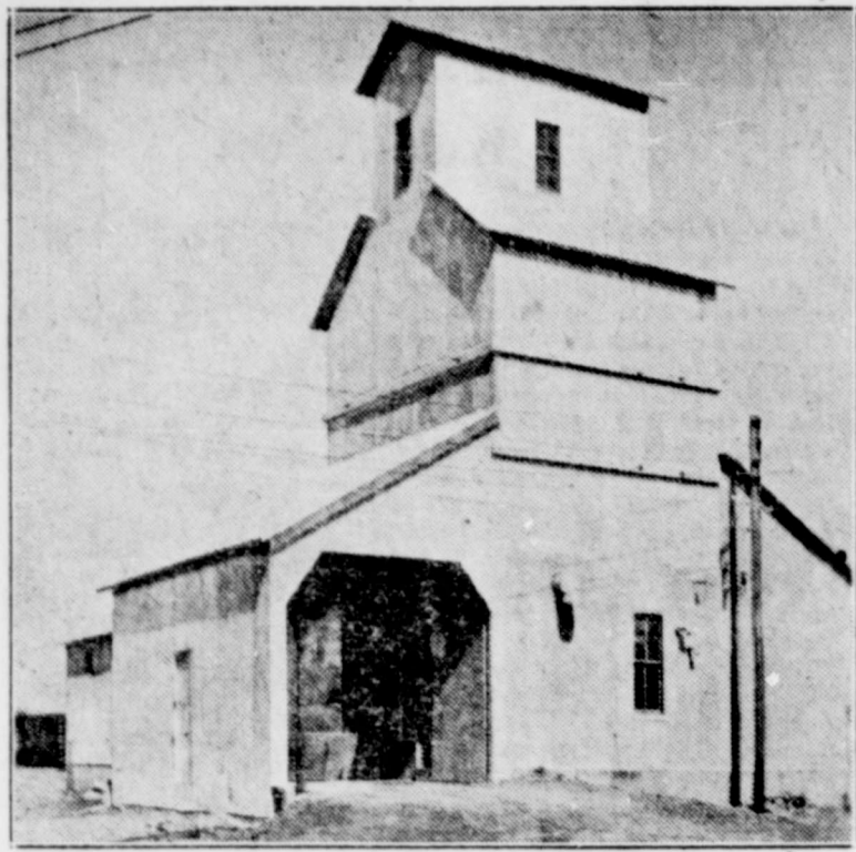
Sudan elevator being overhauled and its capacity doubled. The Company paid the farmers over $300,000 during the past twelve months, and according Manager Payne the Company expects a much larger business during this coming season.
