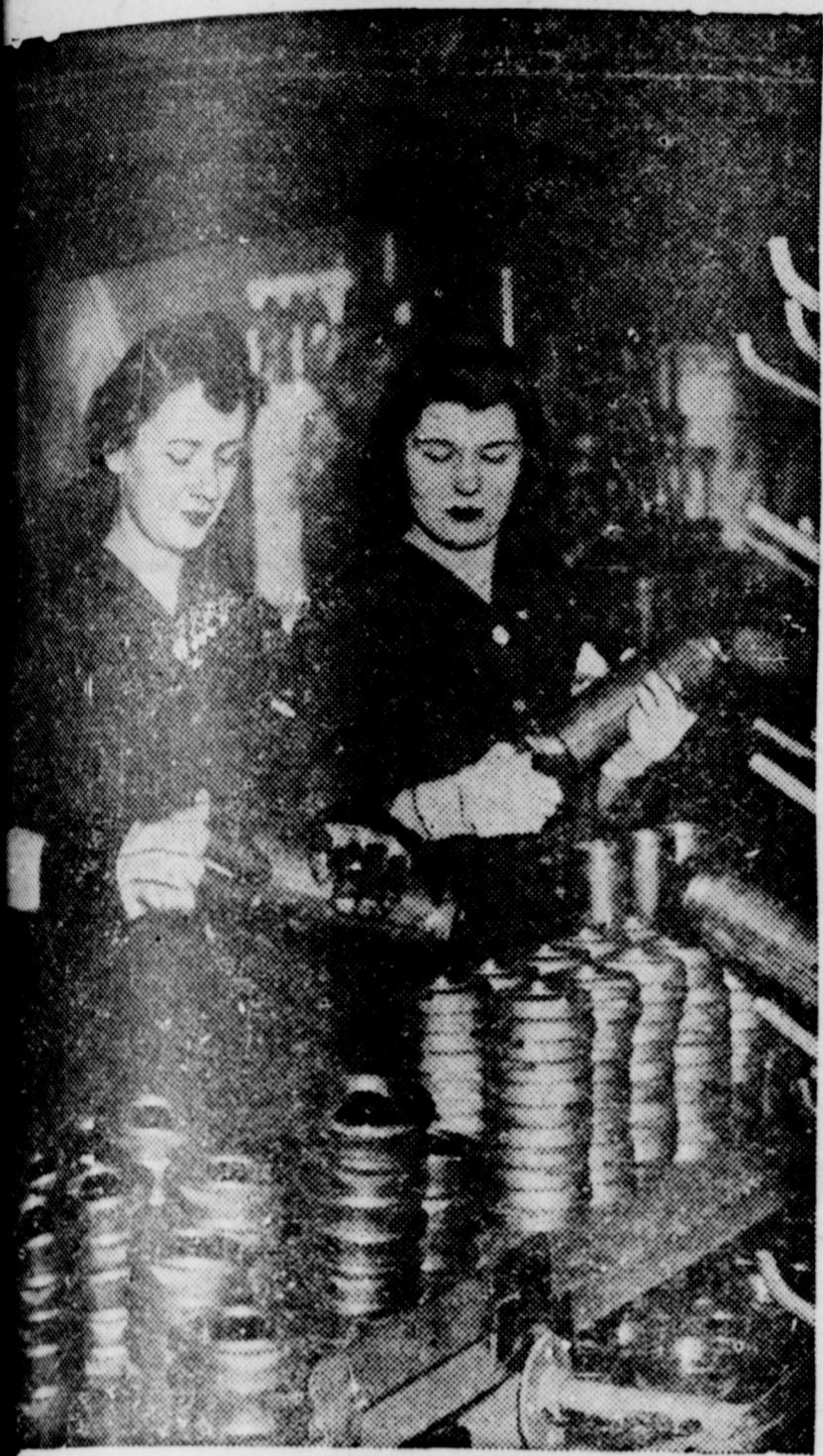
— 2 for men employees of the Budd Manufacturing company, Philadel- are shown putting caps on the new fragmentation bombs being manufactured there for the United States and also for Great Britain. bombs are said to be most powerful of their kind yet developed.
