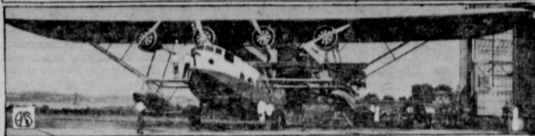
The largest land-and-water airplane ever built, the \$250,000 Sikorsky, has successfully completed its trial flights near Bridgeport, Conn. The amphibian has a wing spread of 114 feet and is engine by four Pratt and Whitney Hornet motors of 575 horsepower. When loaded it will weigh 34,000 pounds. Test flights disclosed that it is handled easily.
