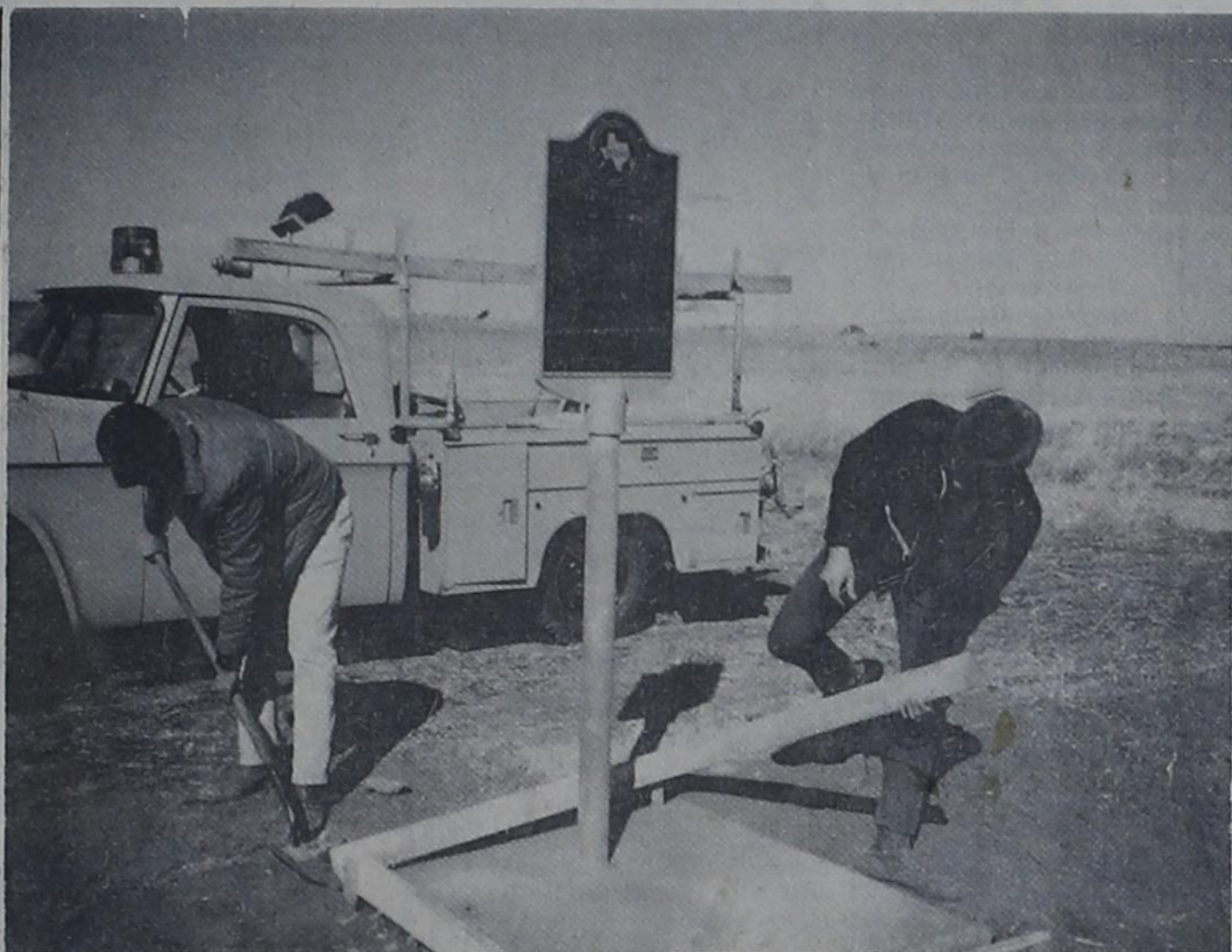
HISTORICAL MARKER --- This new historical marker at the site of the Townsite of Farmerton was installed last week by members of the state highway department crew on Highway 60 between Bovina and Friona. Here, Doyle Wassom, left, and Dean Stovall remove the forms from the concrete base of the marker which is inscribed with history of Farmerton. Founded as Parmer Switch on the Pecos and Northern Railroad in 1898, it was the first county seat of Parmer County and remained so until 1907 when Farwell became the county seat. Dedication ceremonies for the state historical marker will be June 6, announces Hugh Moseley, chairman of Parmer County Historical Society.
