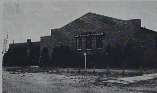
Oklahoma Lane Methodist Church
