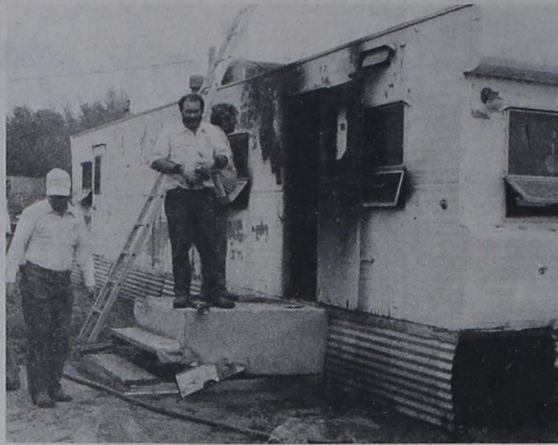
TOTAL LOSS... A fire, apparently started by an electrical appliance in the kitchen area, completely destroyed a mobile home about 3:30 p.m. Wednesday of last week. The mobile home, located in the 300 block of Ninth Street, was owned by Mr. and Mrs. Elton Venable and
