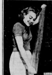
STRETCH" IN GLASS . . . Not pair of hose, but a new plastic 'insides" for safety plate glass s being stretched almost double its length by Miss Wynette Price to show property which imparts resilience and shatter-resistance at all temperatures to new high-
