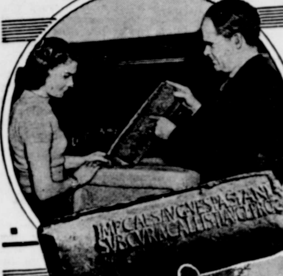
TWO THOUSAND YEARS OLD and still in good condition. A section of lead pipe found beneath the streets of modern Rome is displayed by Director R. P. Show in New York's Museum of Science and Industry. It formed part of the ancient city's water distribution system. Lead pipe is widely used today for this purpose.
