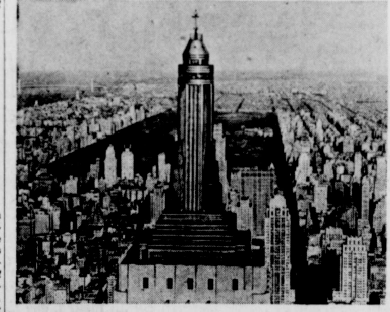
Atop the peak of the world's tallest building, New York's Empire State building, can be seen the new apparatus erected for television broadcasts. Since television waves are not reflected back to earth, they are effective only to the horizon visible from the top of the broadcasting apparatus.
