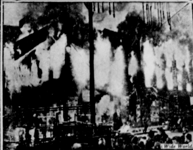
THREE ALARM BLAZE . . . Three alarm mobilization of firemen and fire-fighting apparatus failed to dim this spectacle as flames enveloped upper floors and completely destroyed Philadelphia paper box plant as thousands of persons watched
