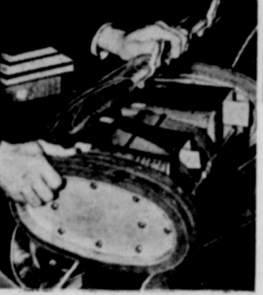
Modernity strikes the staid library of congress. Above: "Speed capsules," a new gadget for shooting books through a 700-foot tunnel in 23 seconds. Their arrival at the destination is cushioned by a bank of air which prevents damage to the books.
