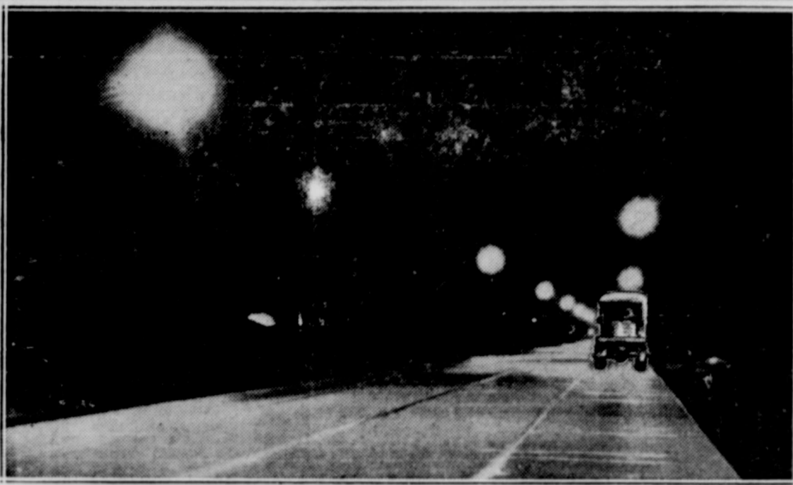
A section of the Skokie Valley Highway, U. S. Route 41, near Northbrook, Illinois, with new modern lights, showing truck and driver clearly visible, five hundred feet ahead.
