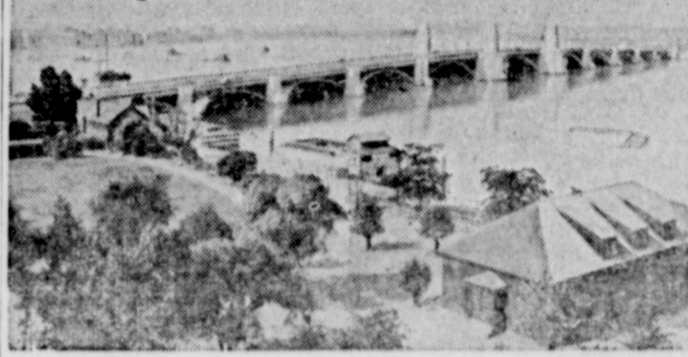
Charles River Basin and West Boston Bridge.
