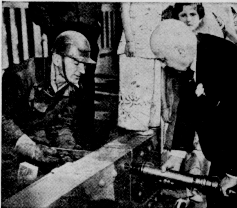
The last rivet was recently driven in the Golden Gate bridge at San Francisco. With many notables witnessing the ceremonies, a crew of iron-hatted riveters drove a golden rivet into the span, signaling completion of the structural steelwork. Mayor Rossi (right) of San Francisco aided by riveter Edward Stanley drives the last rivet.
