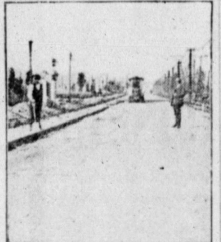
Subgrade Prepared for Concrete Pavement.
