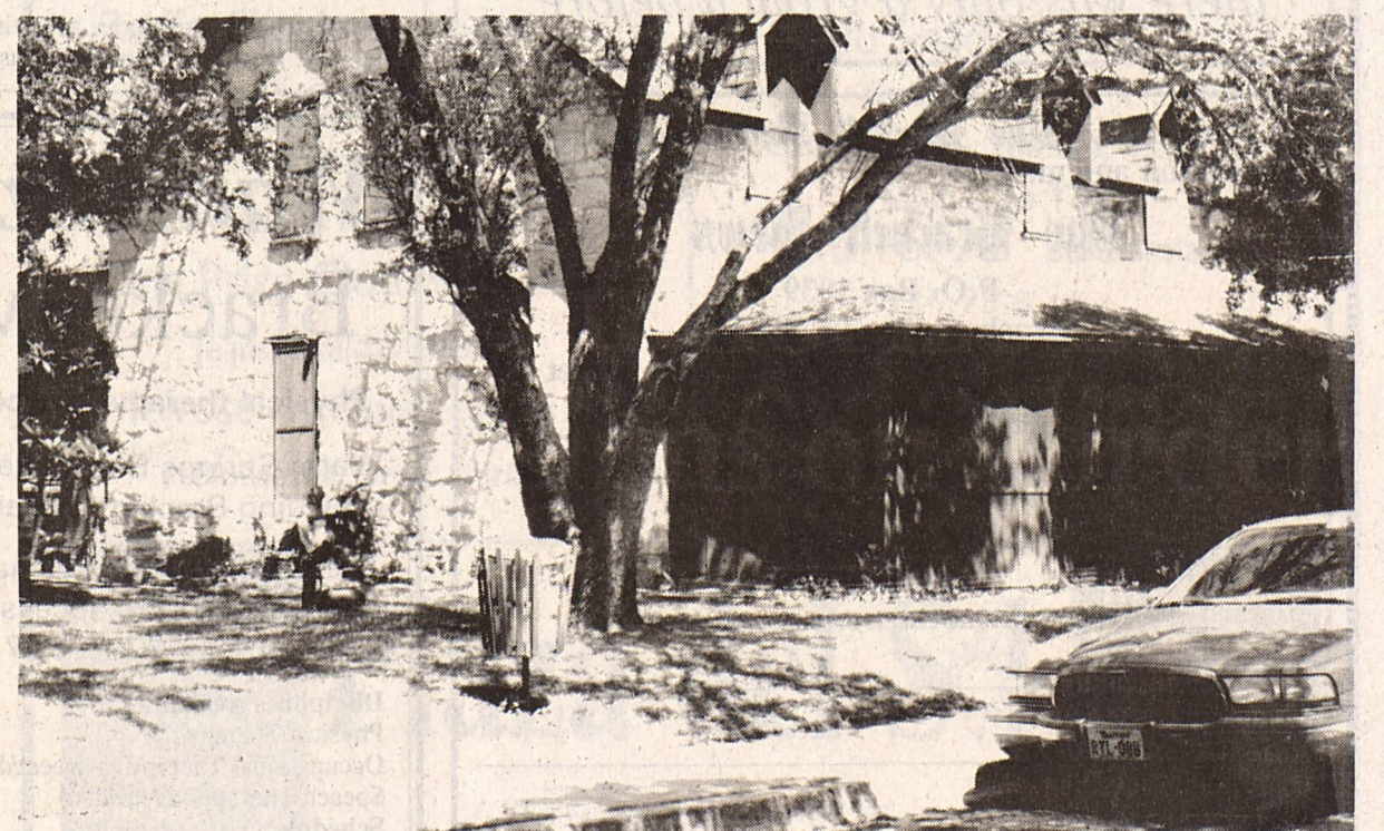
The Shanahan house is one of four homes to be featured in the Kinney County Arts Council's Annual Christmas Tour of Homes on Dec. 13. The house was one of eight designed and constructed in 1874 to accommodate officers' families. Photo Special to The Brackett News
