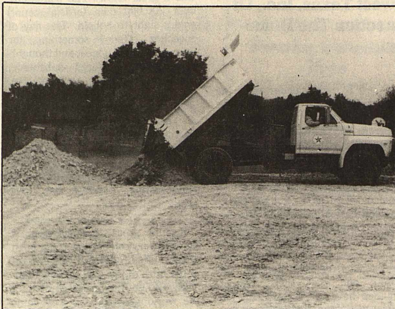
City dump truck dropping a load of dirt on the field.
