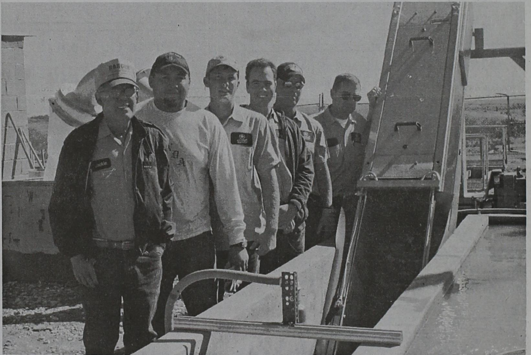
Inspecting the newly installed Automatic Mechanical Bar Screen at the City of Post sewage treatment plant are city staff members (left to right) Jackie Blacklock, Johnny Torres, Brent Justice, John Goin, Dan Nelson and public works director Delbert Rudd. (Photo by Tim Burnett)
