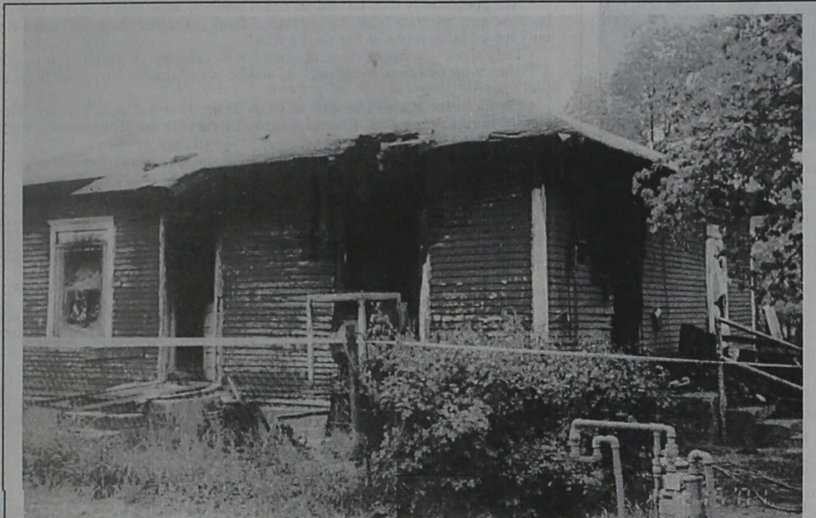
Fire gutted this house on West 10th Street, killing Jose Rodriguez and Gregorio Rodriguez. (Photo by Thomas Zachary)
