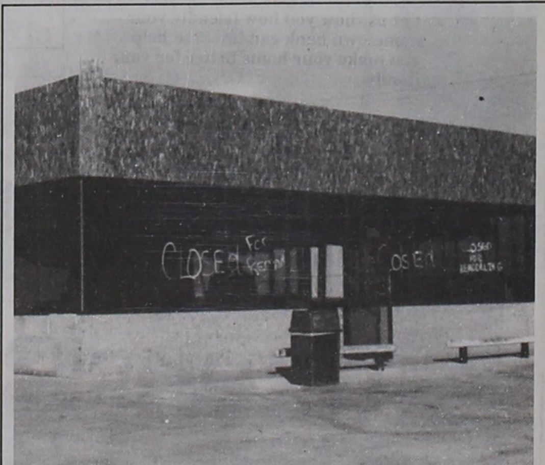
Remodeling at the Post Dairy Queen will take a few more weeks, but when finished will present a new image (see story on Page 2). (Photo by Barbe)
