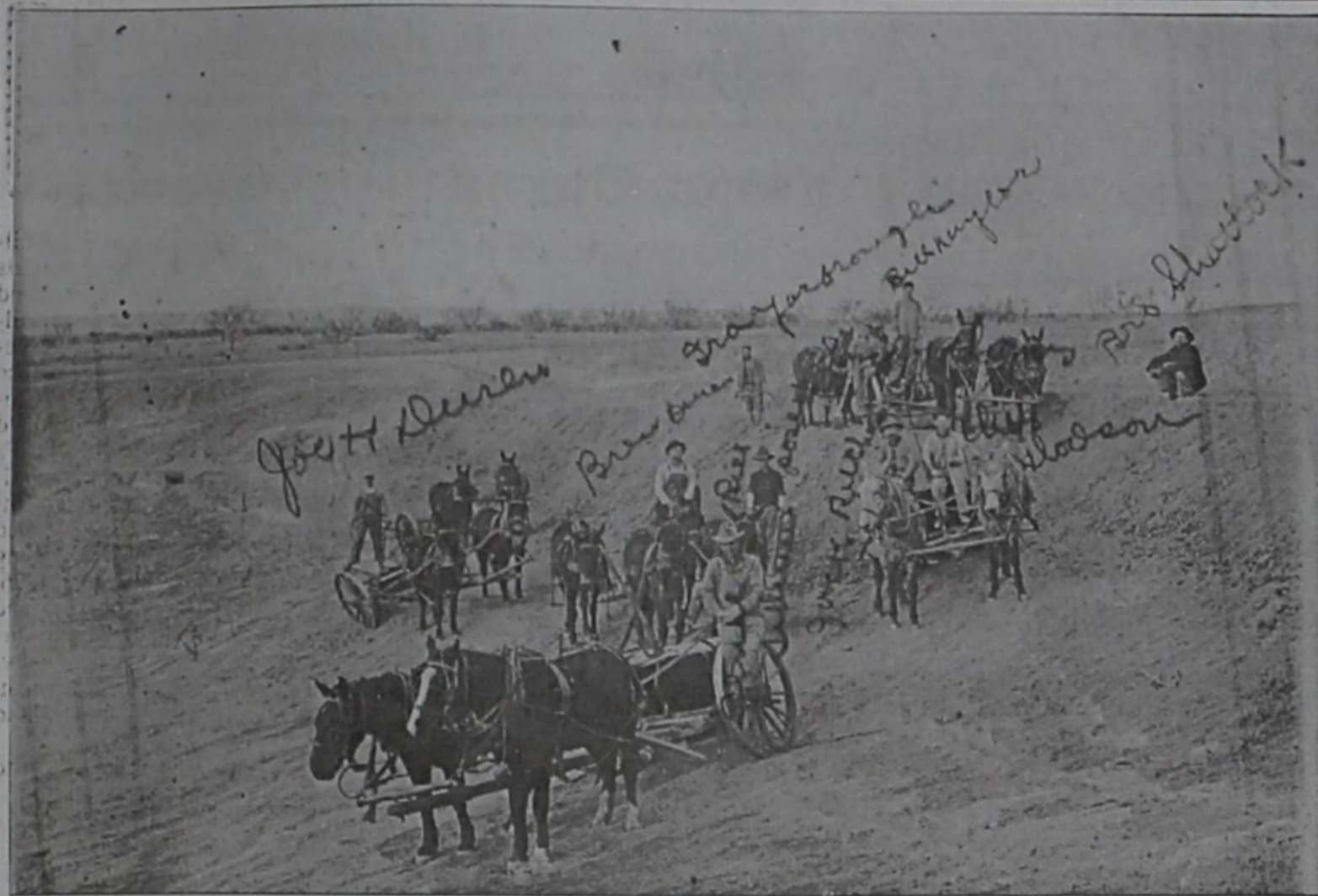
Working with their horses and mules, an early Garza County tank crew scoops out dirt with their "fresnos." Among those in this photo, donated to the Garza County Historical Museum by Bonnie Duren, are Joe H. Duren, Brew Owen, Ira Yarbrough, Bill Naylor, Bro. Shattock, Bill Posey, Jesse (unreadable), Jack Reece and Cliff Dodson. If you are able to provide additional details on this photo, please call the museum at 495-2207.
