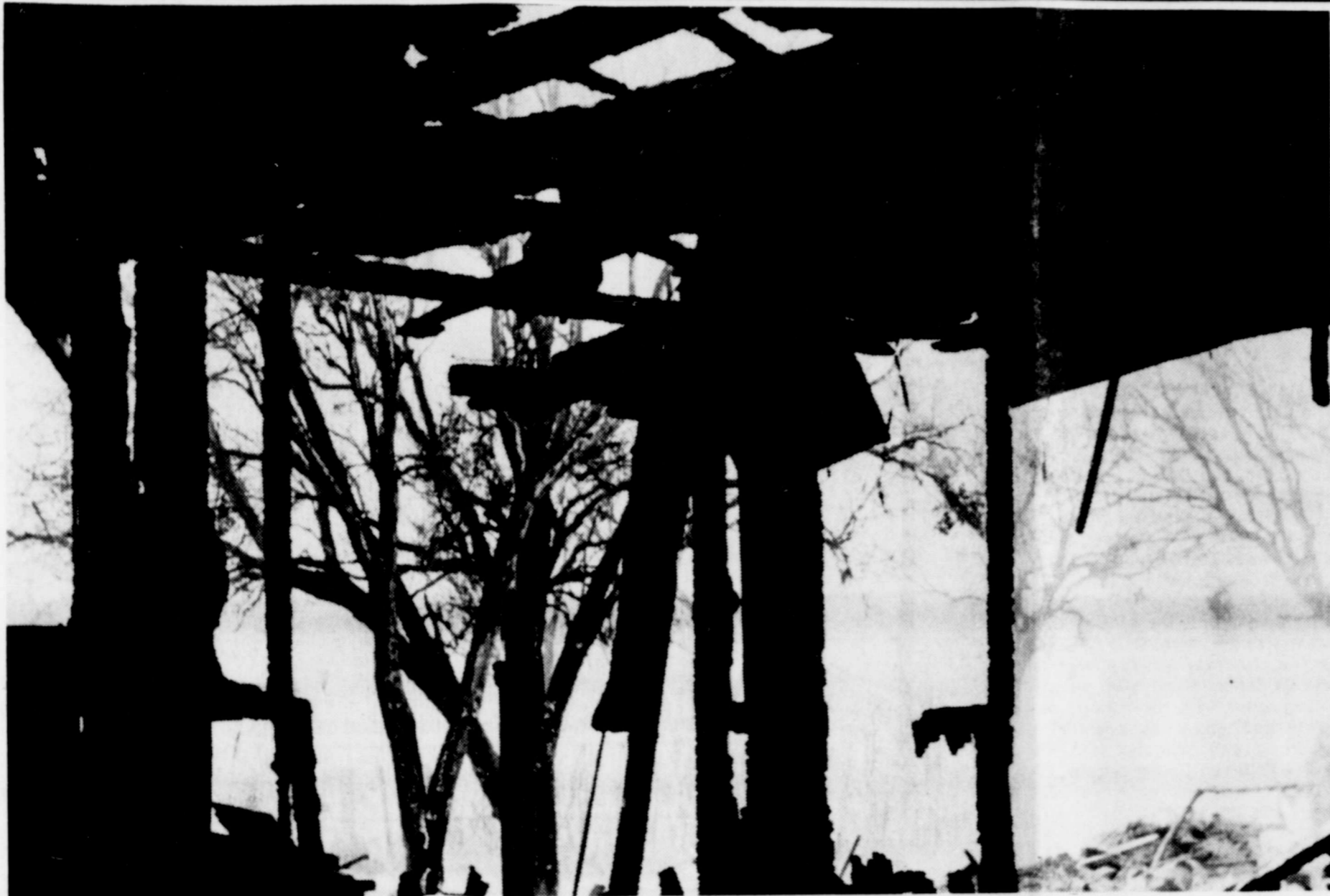
§ The Merkel VFW building was almost completely destroyed by fire here Friday morning.
