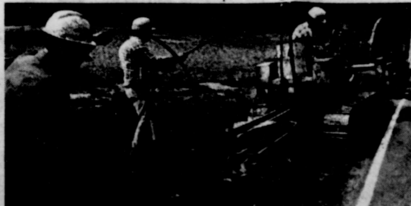
Cable crew working to expand your telephone service
