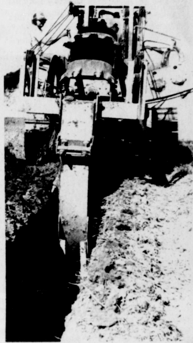
Jerry Cole of Durant, Okla. operates a trencher west of FM 1225 as progress is being made on the Blair Water System. When completed, the system will supply water to 200 rural residents. All of the pipe is on hand in the $480,000 plus project. (Staff photo by Cloy A. Richards)
