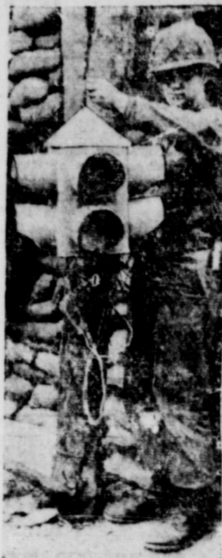
CANNED SAFETY —This "modern" traffic signal will flash its three-way safety signals on a heavily-traveled UN supply route near the Korean front. Made from old food and coffee cans, it gets its illumination from Christmas tree bulbs. Holding it is Pfc. John J. Stingen, of Philadelphia, Pa., who is with the 45th "Thunderbird" Infantry Division.
