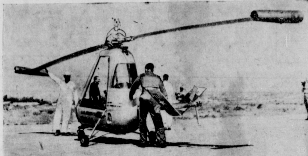
"JEEP" HELICOPTER MAKES ITS BOW —This is the American Helicopter Company's radically new HX-26 helicopter, making its first public appearance at Torrance, Calif. The tiny aluminum craft, weighing less than 300 pounds, is powered by pulse-jet engines at the ends of its rotor blade. Designed for one-man military reconnaissance, the collapsible 'copter can carry more than its own weight at 80 miles per hour.
