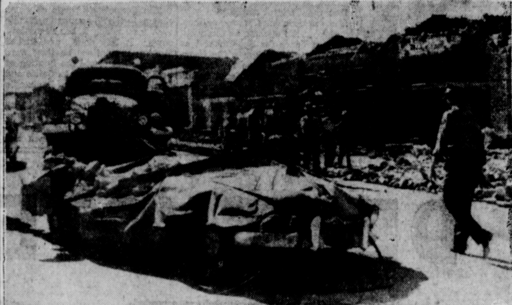
QUAKE SCENE —The main business street of Tehachapi, Calif., lies in ruins from earthquake which shook the little Mojave desert town from its foundations. (NEA Telephone)
