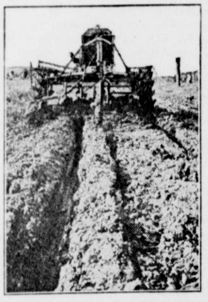
A Modern Machine Working on a Rutty Highway.
