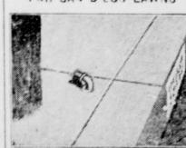
The sidewalks of San Diego, Jan. are equipped, at intervals, with hose connections placed near the curbs, for the convenience of property owners in sprinkling the sidewalk or lawn,-Popular Mechanics Magazine,
