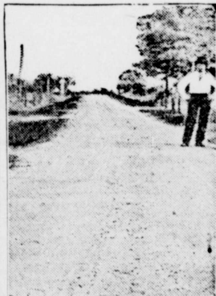
Proper Maintenance Given to This Road.
