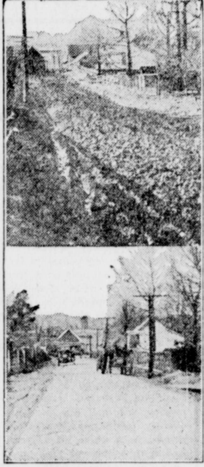
A Country Road Before and After Improvement.
