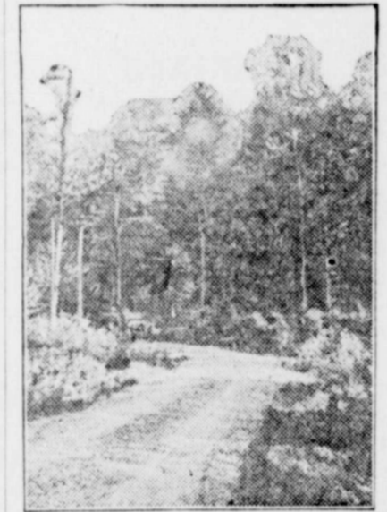
Stretch of Concrete Road in Michigan.
