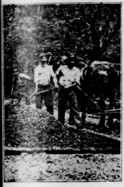
Bituminous Macadam Mixing Method.
