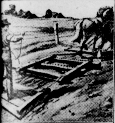
The Spiked Forward Part of the Drag Loosens the Road Soil, and the Following Rear Portion Packs It to a Smooth Surface, Thus Finishing the Surface in One Operation.
