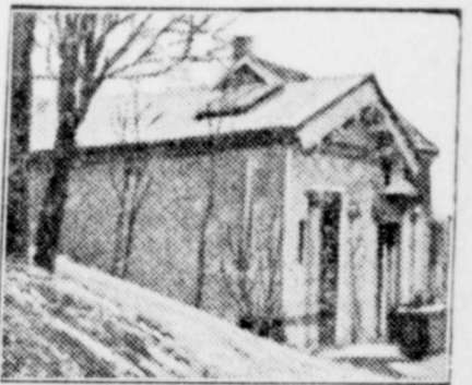
Side View of the Dwelling: In This Picture Can Be Seen the Frame Portion of the Structure, Which is Scarcely Visible From the Street.
