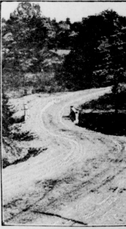
Asphalt Binder Road.
