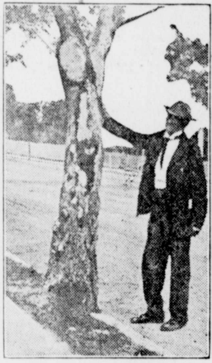
Putting a new heart into a tree. Cement has been substituted for the "heart" and most of the body.
