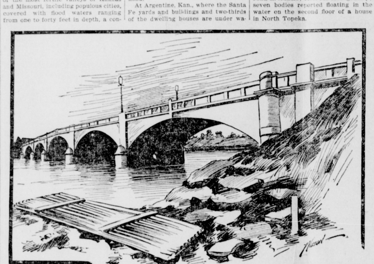
Bridge Over Kansas River From North Topeka Side.
