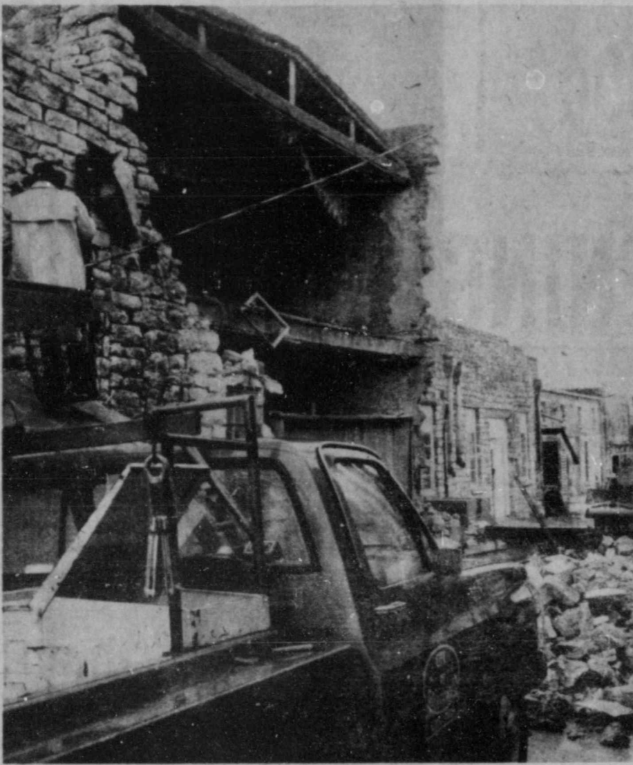
Old Building Wall Collapses
