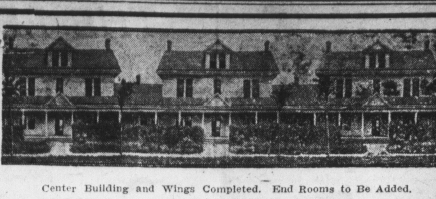
Center Building and Wings Completed. End Rooms to Be Added.
