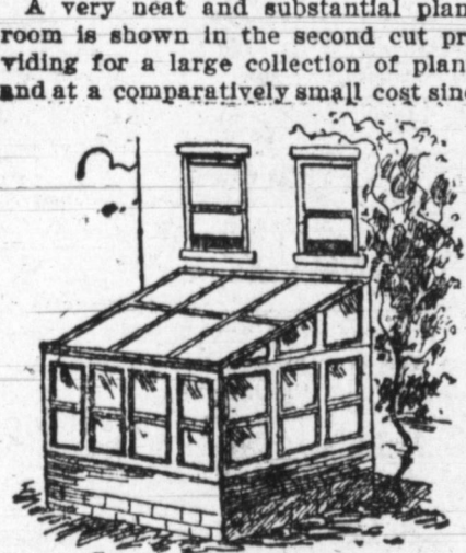
GREENHOUSE ADDED TO DWELLING.
