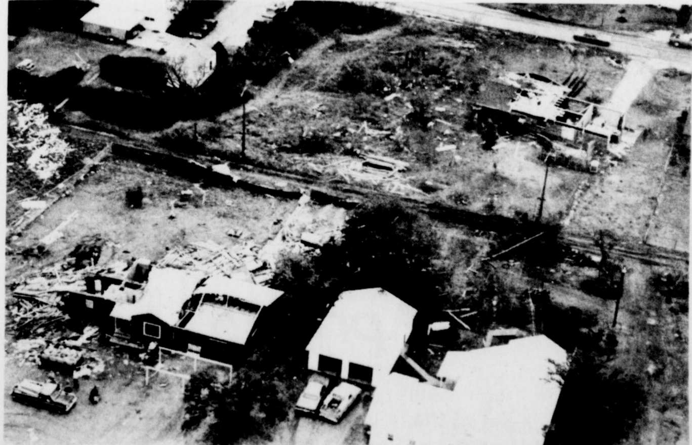
AN AERIAL LOOK —This aerial view of the northeast part of Crowell shows two homes which were completely demolished when a tornado ripped its way through the town at 2:07 a. m. Saturday. The Fred Adcock home's roof (background) was removed and blown through the home of the Jimmy Hudgens family, foreground, as the tornado moved northeastward, leaving more than 30 homes and businesses heavily damaged or destroyed and an estimate of at least $175,000 damage to the city. (Aerial photo by J. T. Smith and Marvin Machac. Courtesy Abilene Reporter-News.)
