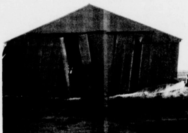
DAMAGED IN THURSDAY WIND —This barn on the farm of Mrs. Roy Ayers in the Riverside community, suffered heavy damage in a tornado which skipped across that part of the county late Thursday, more than a day before the tornado damaged Crowell early Saturday morning. Another small barn at the Ayers farm was also damaged.
