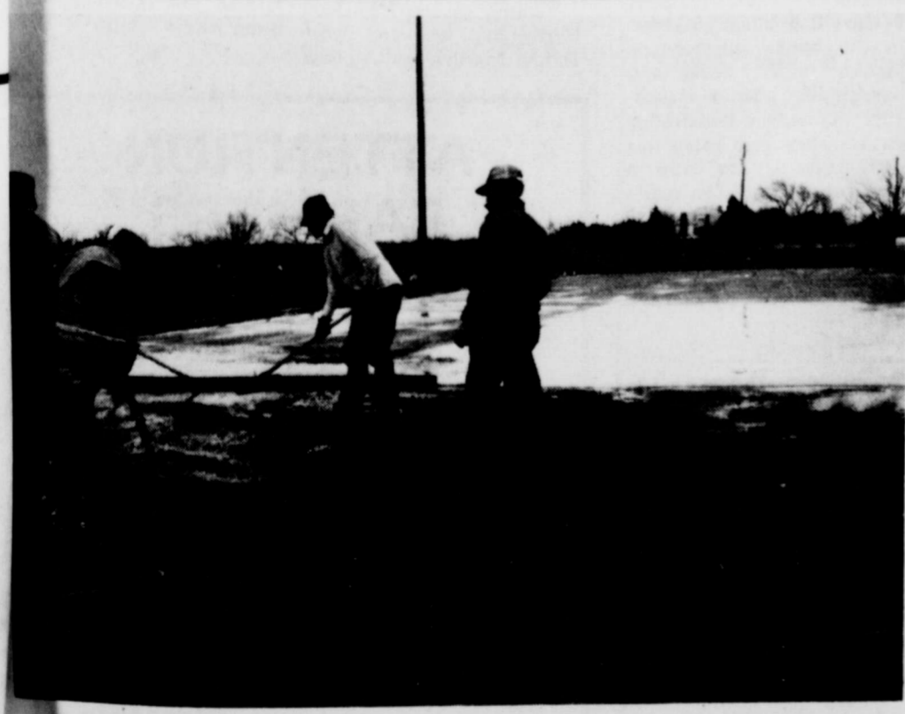
AG PAVILION FLOOR FINISHED —This picture was made last Friday morning as the last load of cement was poured on the floor of the new Crowell Ag Pavilion. The picture is looking east and shows the fresh 40x100 foot section just poured. To the right, out of the picture, is the other
