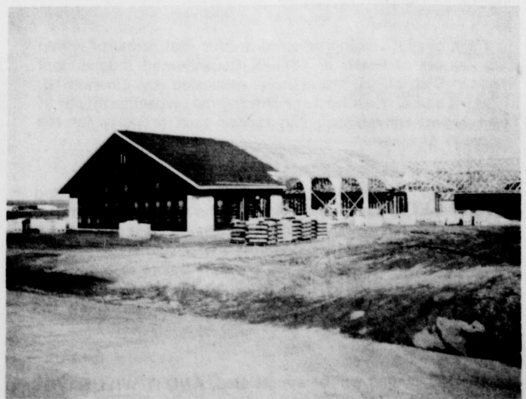
Work Progressing on New First Baptist Church Building
