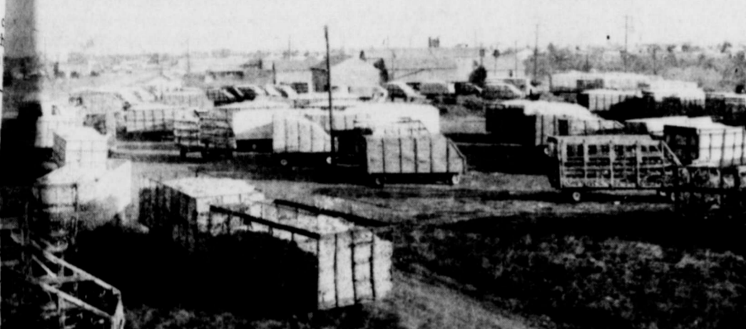
LOTS OF COTTON --This view looking north at the Farmers Co-Op. Gin in Crowell shows so literally hundreds of bales of cotton waiting to be ginned. The county's three gins have been swamped like this for several weeks and there is still lots of cotton to be gathered. This photo was made last Friday morning.
