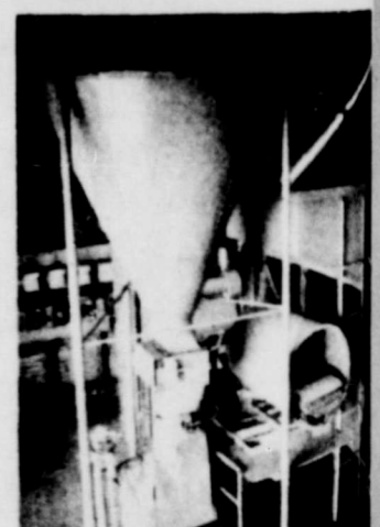
All-automatically controlled bagger
