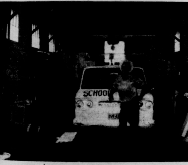
OLD BUS SHOP —Allen Taylor, school employee, is shown above standing in the old bus shop, which will be replaced by the new building under construction. (News photo)
